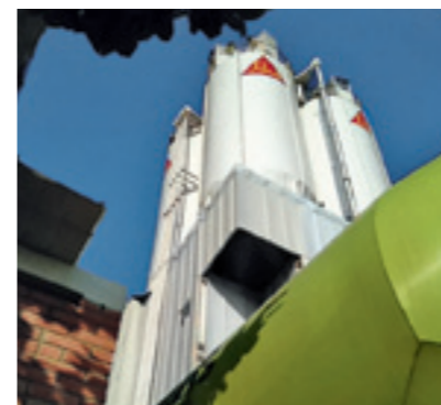
RAINWATER BASED PRODUCTION, SIKA COLOMBIA PLANT BARRANQUILLA, COLOMBIA
