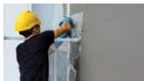
Building Finishing / Dokončovanie stavieb
