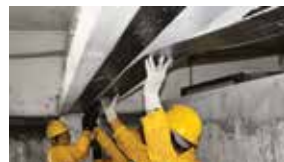
Refurbishment / Oprava a ochrana betónu
