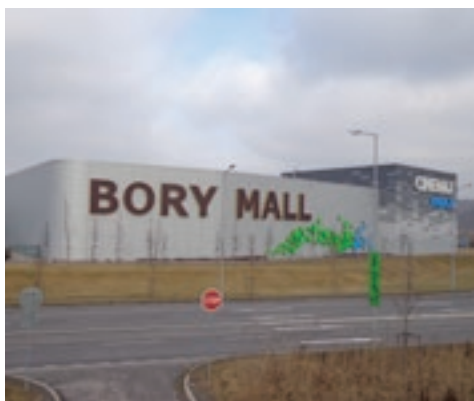
Bory Mall, Bratislava, Sika CarDeck systémy – 18.000 m 2
